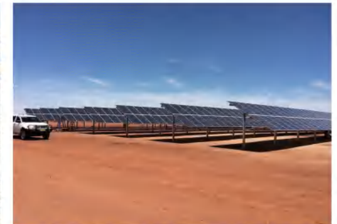
Steel Ground mounting in Australia
