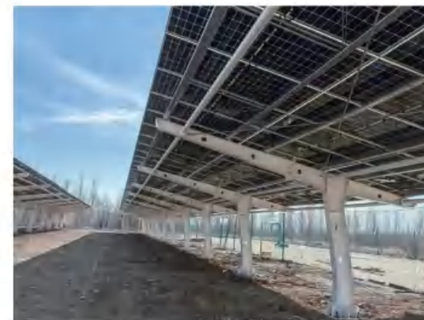
Steel carport in China
